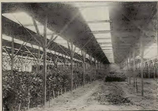
Fig. B. Interior view, showing construction. Shed erected by G. I. Taber, Glen Saint Mary Fla.
